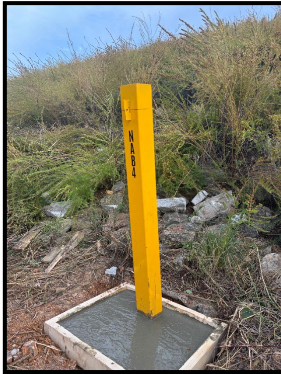
Photograph 9: View of repaired well pad, re-painted and re-labeled stickup at NAB-4.
