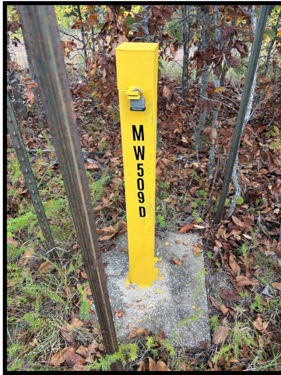
Photograph 5: View of re-painted and re-labeled stickup at MW-509D.
