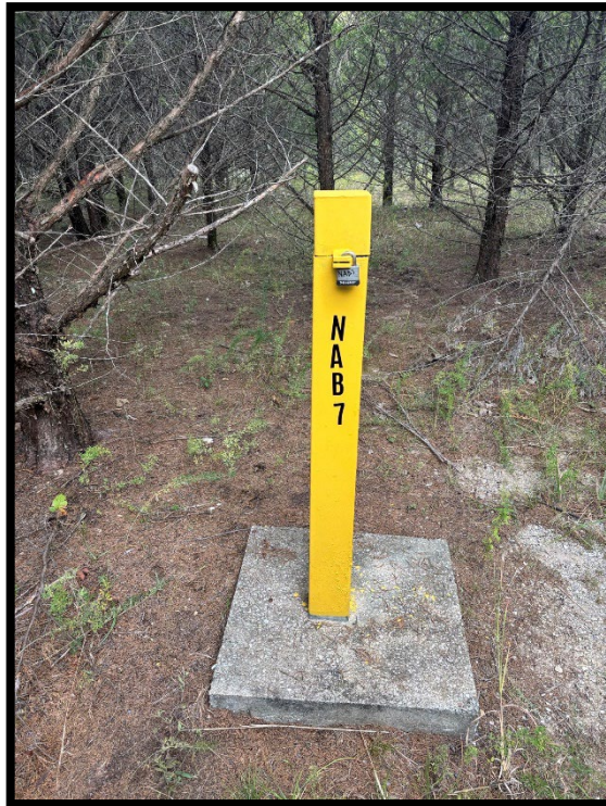
Photograph 10: View of re-painted and re-labeled stickup at NAB-7.
