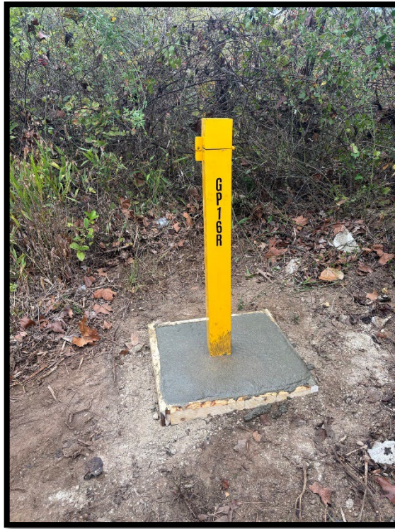
Photograph 11: View repaired well pad, re-labeled and re-painted stickup at GP-16R.
